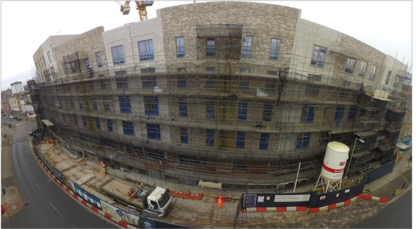
Figure 3 View towards the High Street elevation
